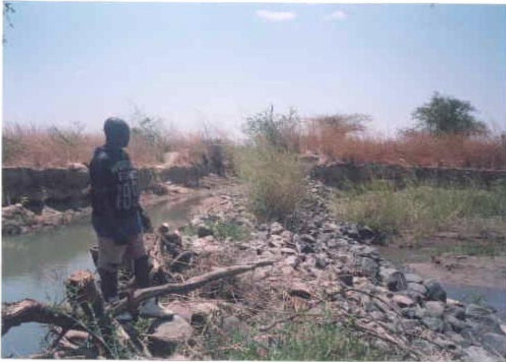
Plate 1: Stone intake at Isenyela Furrow, Kimani River
